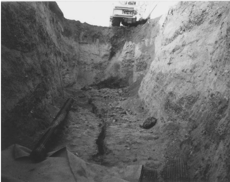
Figure 3.40 Reactivated fault exposed in a trench on Downes Bank. The trace of the fault is marked by a ground fissure about 0.1 m wide. Remediation of the fault was to be made using a geotextile mat and granular fill.
