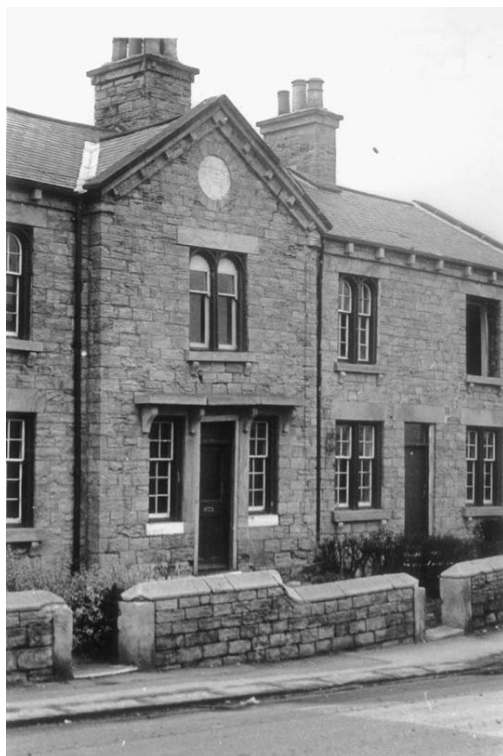
Figure 3.11 Subsidence damage in the neighbourhood of a fault step (windows fell out, door frames twisted and masonry severely cracked) Elsecarr, South Yorkshire, England. Fault step corresponds with dip in road.
