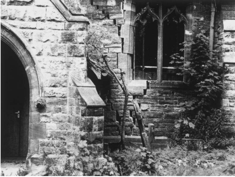
Figure 3.35 Damage to Barlaston Church caused by fault reactivation at a sandstone-mudstone contact.
