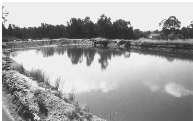
Figure 8.15 Pollution control pond, one of four.
