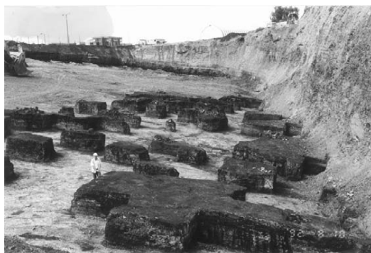
Figure 2.1a Old pillared workings in coal exposed at the Tinsley Park opencast site, Sheffield, England.
