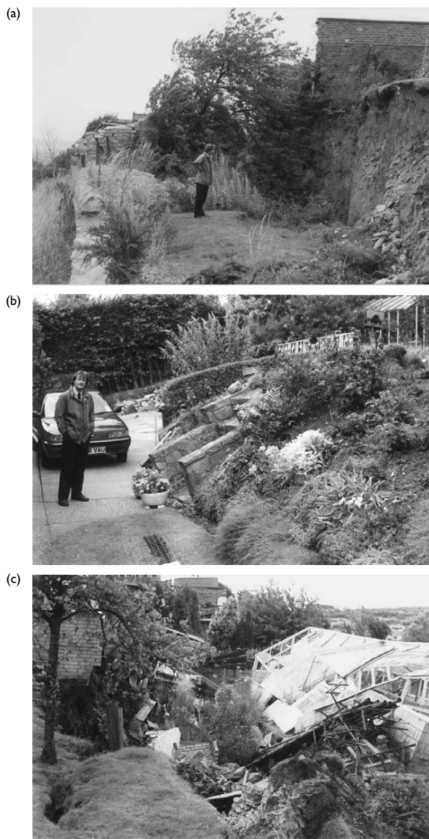
Figure 10.17 (a) The backscarp of the mining-induced landslide at Bolsover, Derbyshire, England. (b) The upheaved toe of the landslide at Bolsover, now landscaped. (c) Structural damage to a perimeter garden wall and a greenhouse at the crest of the Bolsover landslide.
