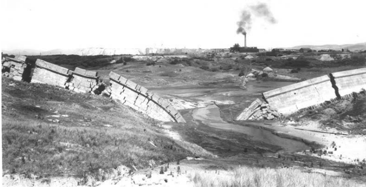
Figure 4.6 Subsidence, up to 20 m in places, above Hodbarrow Mine, Millom, Cumbria. (Reproduced by kind permission of the British Geological Survey. © NERC. All rights reserved. IPR/61–05C.)
