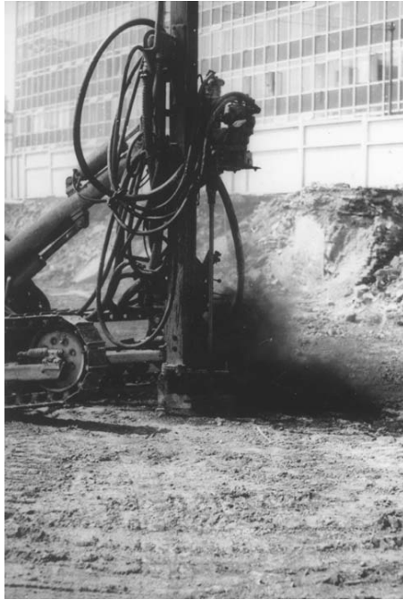
Figure 2.16 Probing for shallow old mine workings in coal with a rotary percussion rig, Sheffield, England.
