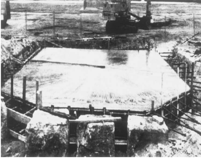
Figure 2.27 Heavy duty reinforced concrete slab acting as a cover for an old mine shaft. (Reproduced by kind permission of White Young Green Consulting Limited, International Mining Consultants Limited and the Coal Authority.)
