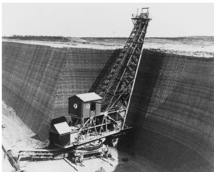
Figure 6.18 Working the Oxford Clay with a bucket-chain excavator for brick making at Whittlesey, near Peterborough, England.
