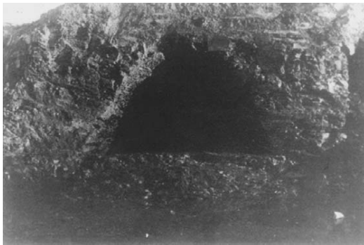
Figure 2.2a A bell pit working in an ironstone band revealed by opencasting at Sproats site, Northumberland, England.
