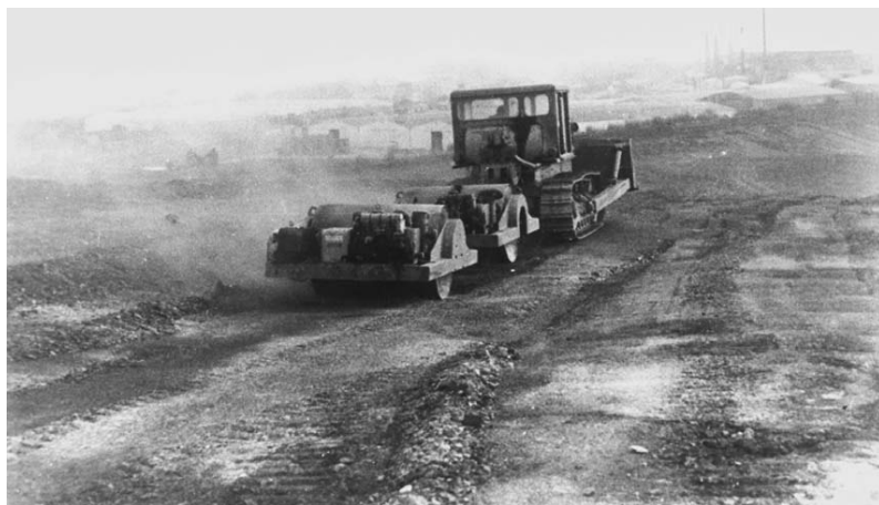
Figure 7.14 Compacting spoil with a vibratory roller.
