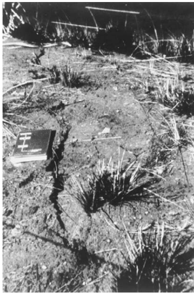
Figure 4.25 Cracks developed on the north bank of the M2 motorway due to subsidence.
