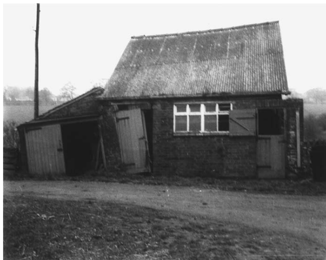
Figure 5.18b Severe damage caused to farm buildings due to subsidence caused by the abstraction of salt brine, Cheshire, England.
