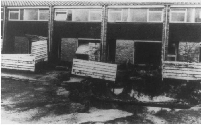
Figure 2.7 Collapse of shallow workings in chalk at Jacqueline Close, Bury St Edmunds, Suffolk, England, the Close ultimately was abandoned.
