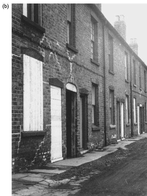
Figure 3.2 Examples of subsidence damage due to longwall mining of coal, Elsecarr, South Yorkshire, England, showing extensive cracking, walls being shored, and doors and windows blocked up after frames being severely twisted.
